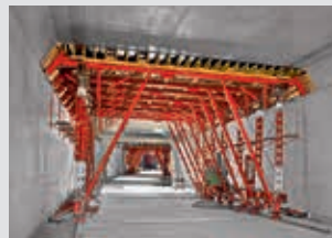
Tunnel Formwork
